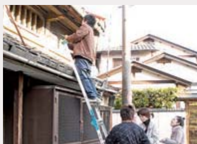
▲ Survey of a traditional building
